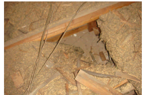
Void /lacking insulation over the kitchen.
