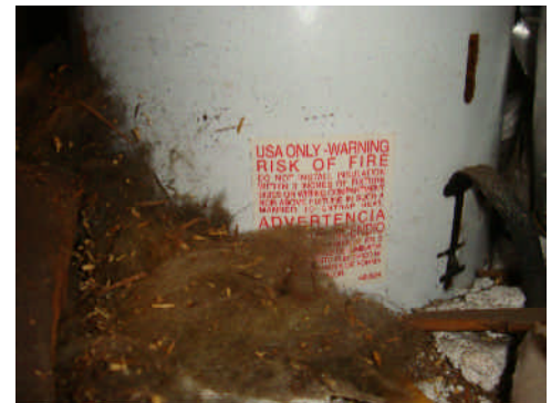
Void /lacking insulation over the kitchen.
